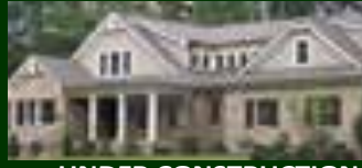
UNDER CONSTRUCTION 32714 Waxberry 4 Bed, 3 Bath, Bonus Rm, Cul-de-sac $435,000
