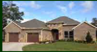
32715 Waxberry Under Construction 3 Bedrooms, 2 1/2 Baths Cul-de-sac Street
