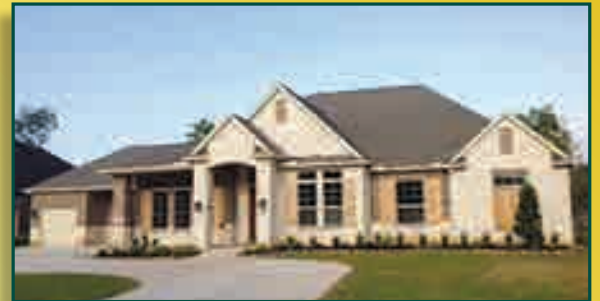
Custom Home being built on our client's lot in Weston Lakes
