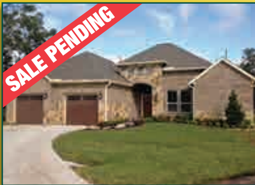
32715 Waxberry - under construction 3 Bedrooms, 2-1/2 Baths Cul-de-sac Street
